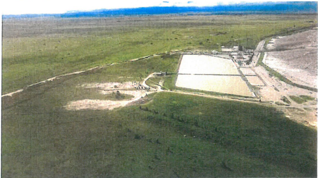
Figure 2: Spillage towards the Vaal River (21 Feb 2017)
